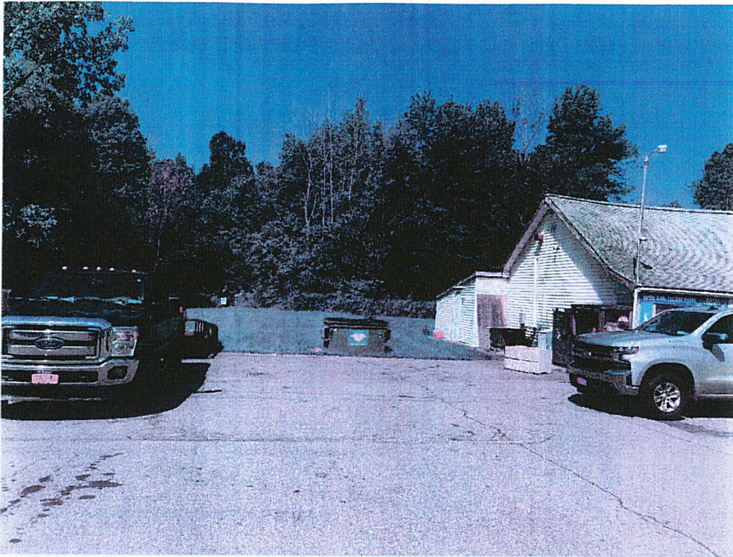
3. South side of building
