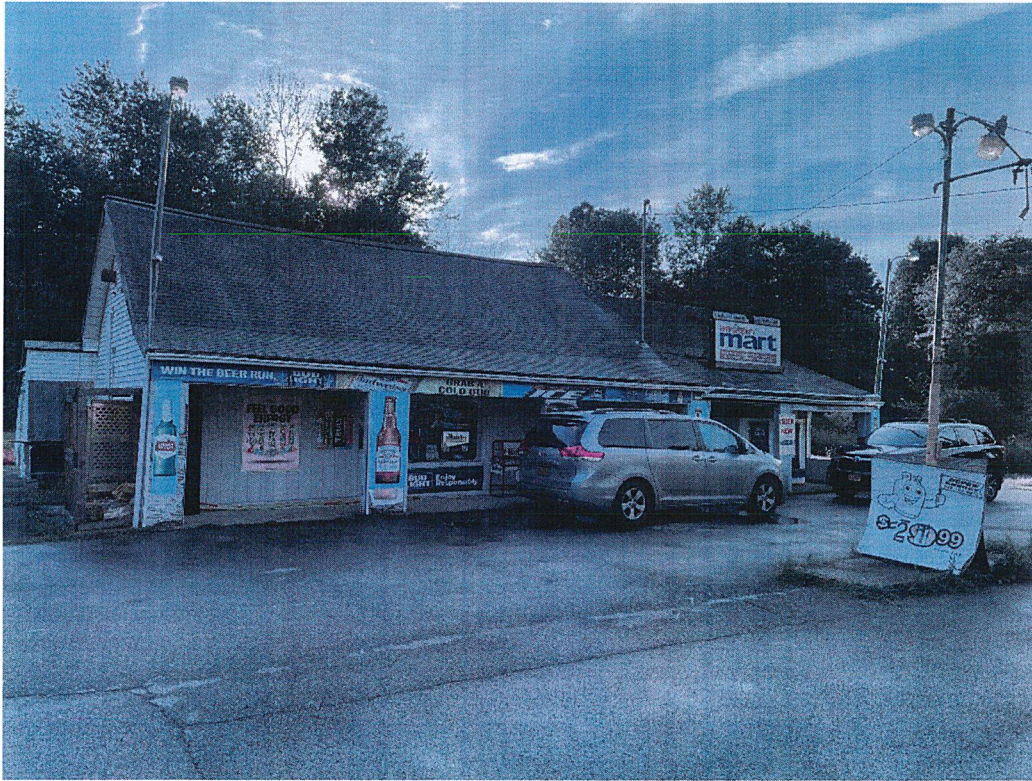
1. Front of Building (looking west)
