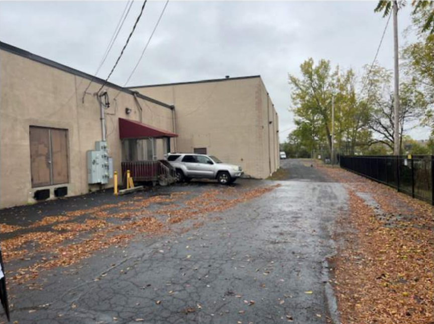
EXISTING EXTERIOR LIGHT
