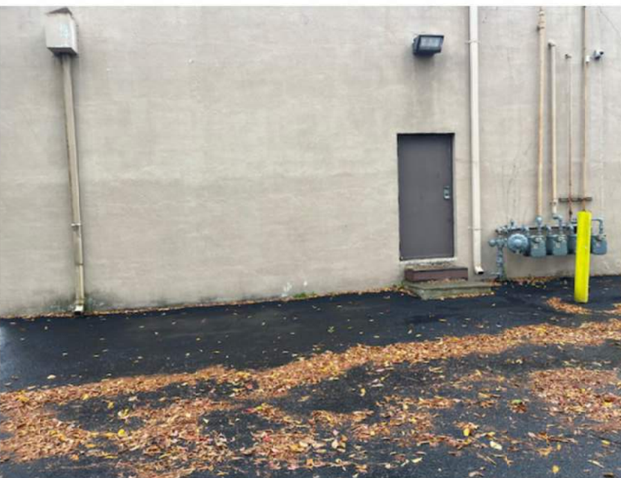
EXISTING EXTERIOR LIGHT
